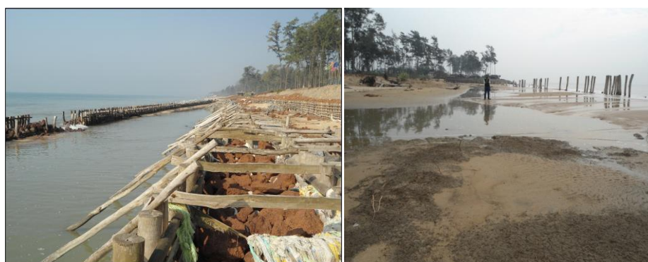
Photo No-1 : Narrowing beach width and exposed mud bottom along the chandpore coast
